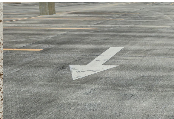
Construction of traffic and parking areas
